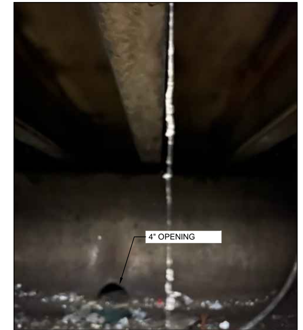
H - 4" DRAINAGE OPENINGS IN LOAD CELL - FOOTINGS INSIDE OF SCALE PIT
