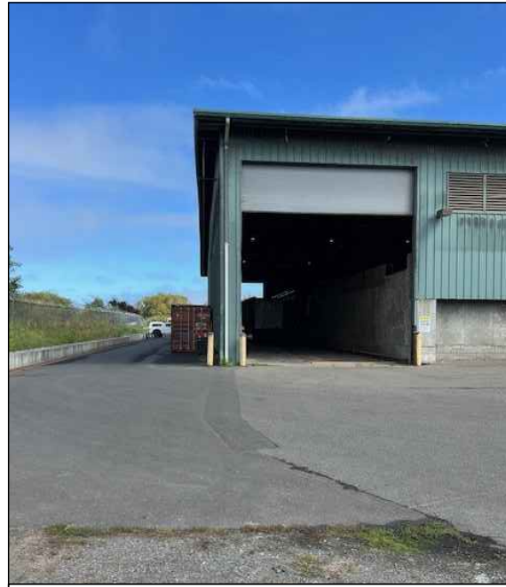
A - OUTSIDE TRANSFER BUILDING - LOOKING NORTH
